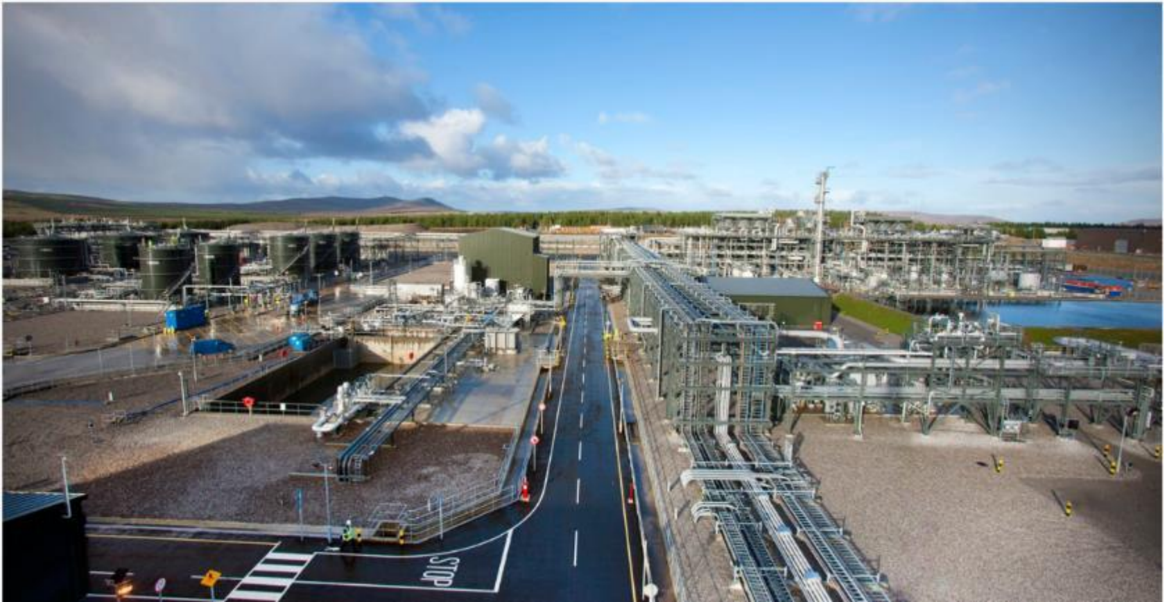
Bellanaboy Bridge gas terminal, photo courtesy Shell Ireland
